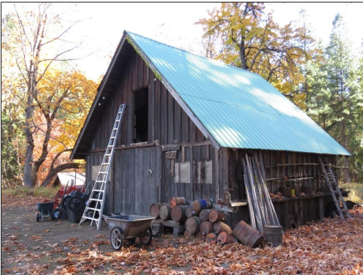
Replacement of the shop's metal roof
