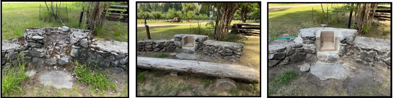
YARD FIREPLACE STABILIZATION AND RESTORATION
